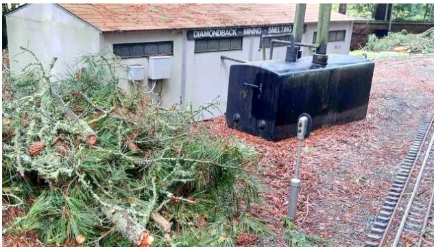
Piles of debris from a pine tree damaged two years ago near the Diamond Back Mine were finally removed
